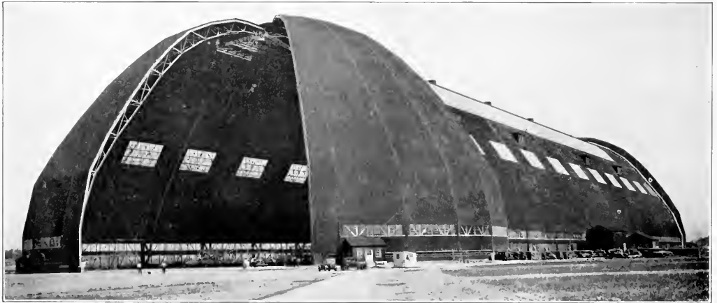
The Goodyear-Zeppelin Corporation airship factory and dock at Akron, Ohio. This building has the largest uninterrupted floor space of any yet constructed—364,000 square feet, or approximately eight acres. Its length is 1175 feet between center lines of door tracks; its width is 325 feet; and its height from floor to the top is 211 feet. A similar dock is being built at Sunnyvale, California.
